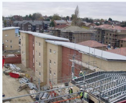
Metek roof trusses to accept Metek roof panel - works in progress
