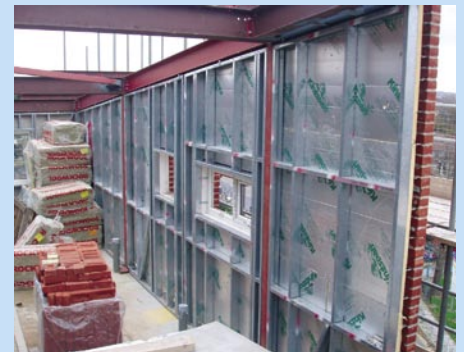
Metek light steel external envelope high-level infill
