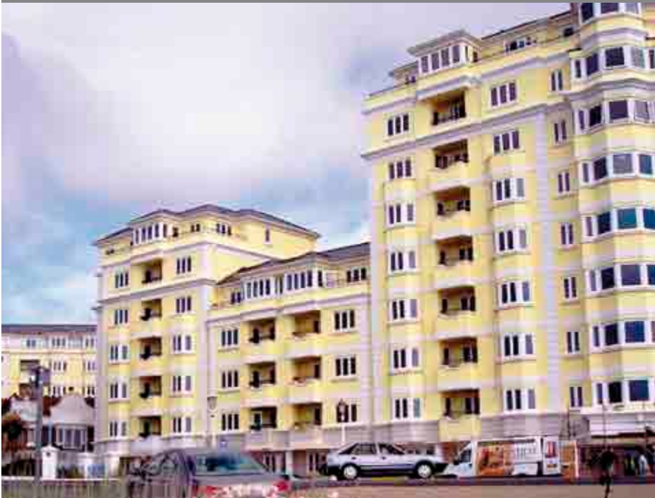
Berkeley Homes' Devonshire Court development at Eastbourne
