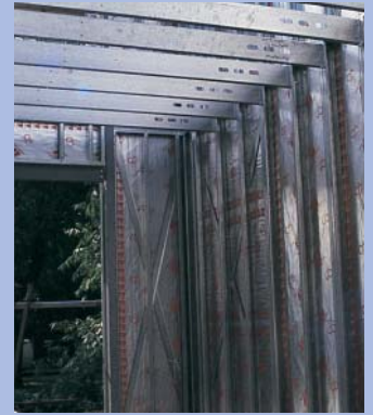
Bolted structure is erected quickly.
