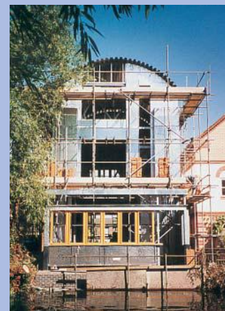
Construction viewed from the riverside.
