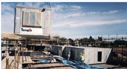
Individual modules are craned onto previously prepared foundations
