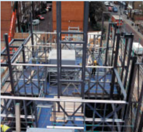
Installation of light steel frames
