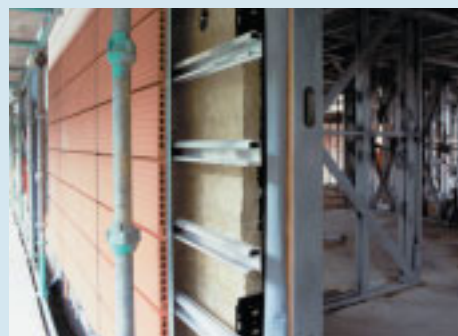
'Rain-screen' cladding during installation
