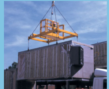
Modules being lifted into place (using man-basket)
