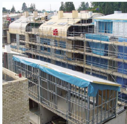
Aerial view of Metek's light steel framing – works in progress
