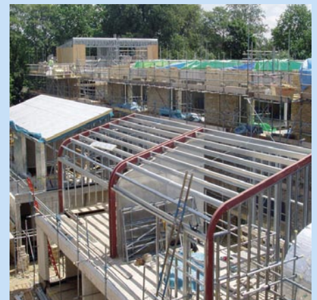
Metek Annexe design with hot rolled curved sections
